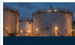
Oil Tank Area
